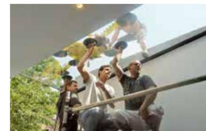
**GLAZED CEILING** Frameless glass panels were lifted over the house with a crane and manoeuvred into position
