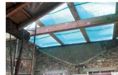
**NEW ROOF** A mono-pitch roof frame was constructed, giving the first floor much higher ceilings for a brighter, more spacious feel
